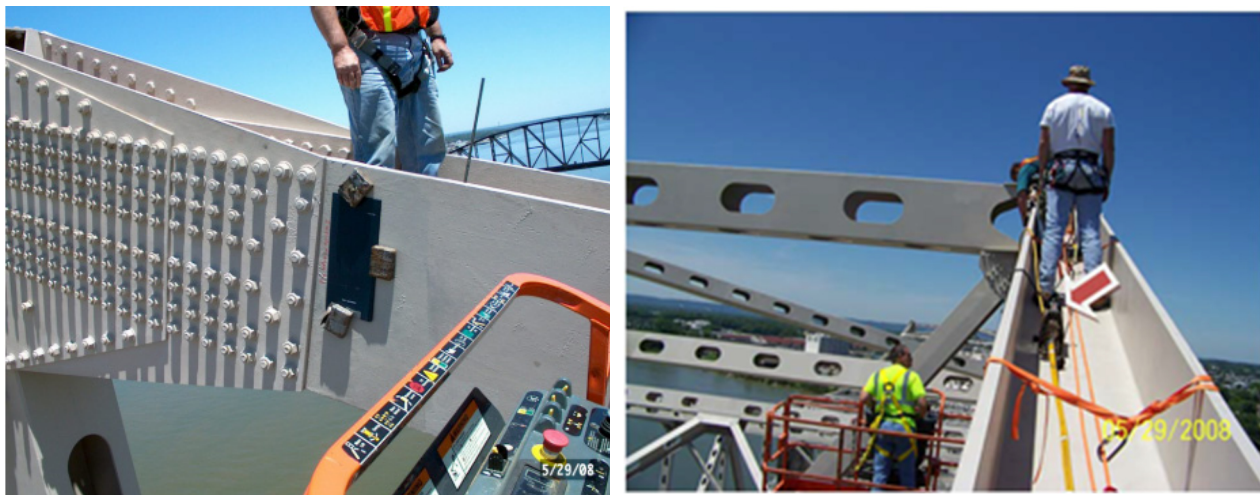
Figure 1-18 Inspection of a steel element using RT Method [3]
