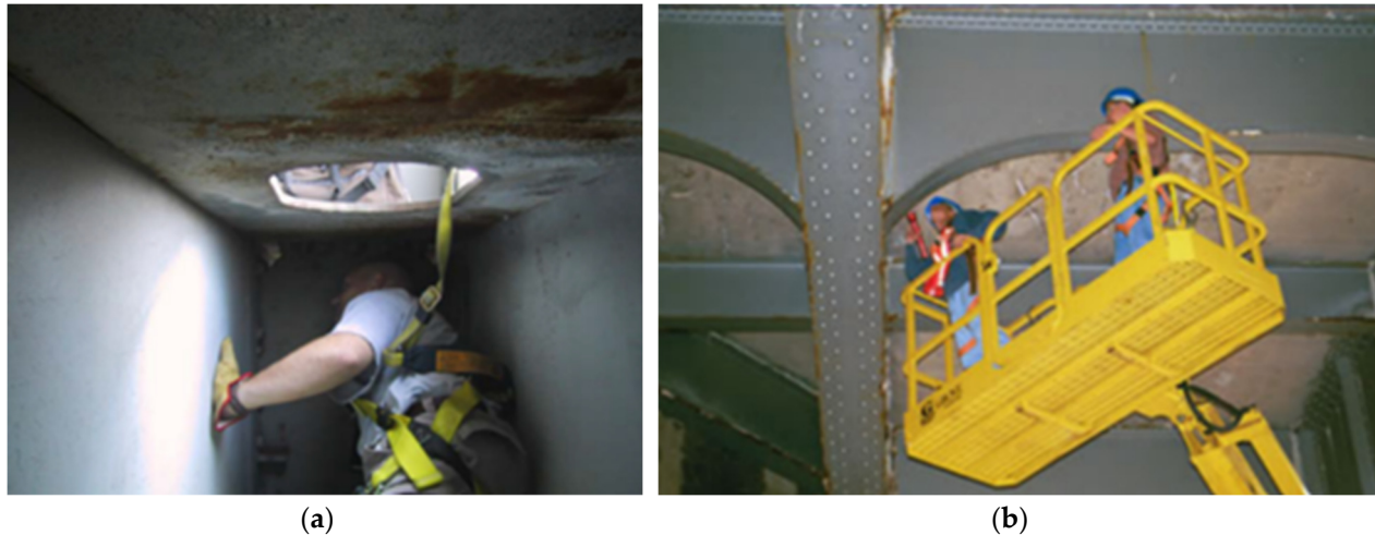
Figure 1-1 Challenges of visual inspection method: (a) Lack of lighting [3]; (b) Visual inspection at heights can be dangerous and challenging [1]
