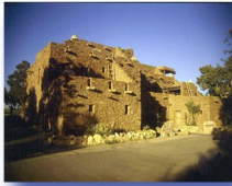
1905 Hopi House, Grand Canyon Village, Arizona, USA
