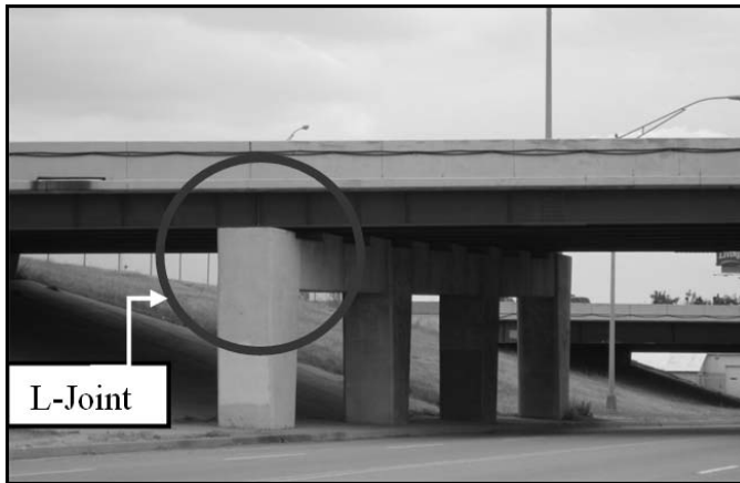
(a) L-joint of bent cap of I-35 overpass in Oklahoma City, OK
