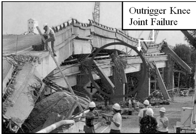
Figure 1-2: Collapse due to outrigger knee joint failure during 1989 Loma Prieta Earthquake (Wikipedia, fn. USGS)
